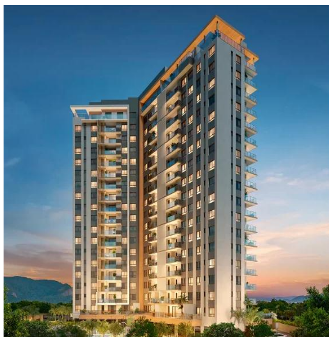
Patrimar | Epic Golf Residence, Rio de Janeiro/ RJ Launched – 2Q25
