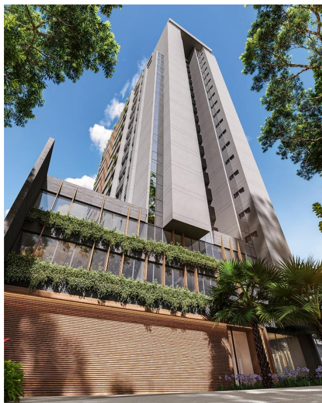
Patrimar | RJ 2300 – Belo Horizonte, MG Delivered 1T25
